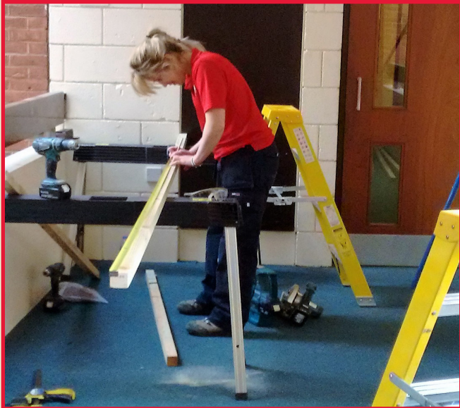
Above: Claire installing low-energy lighting throughout Sorrel and Campion House.
