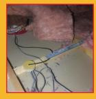
A tenant had installed some downlights but the fittings were non-fire rated and covered in metal sweet tins. The cables were also poorly jointed, posing a fire risk.
