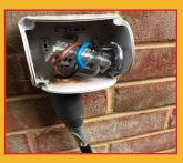
A tenant had installed a hot tub in their rear garden, connected into the cooker switch to provide a supply.
